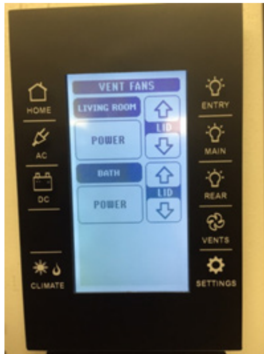
Figure VIII Remote Vent Fan Operating System
