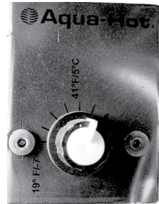
Aqua-Hot Thermostat (located behind service panel) It is factory preset and should not require adjustment.
