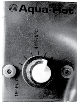
Aqua-Hot Thermostat (located behind service panel) It is factory preset and should
